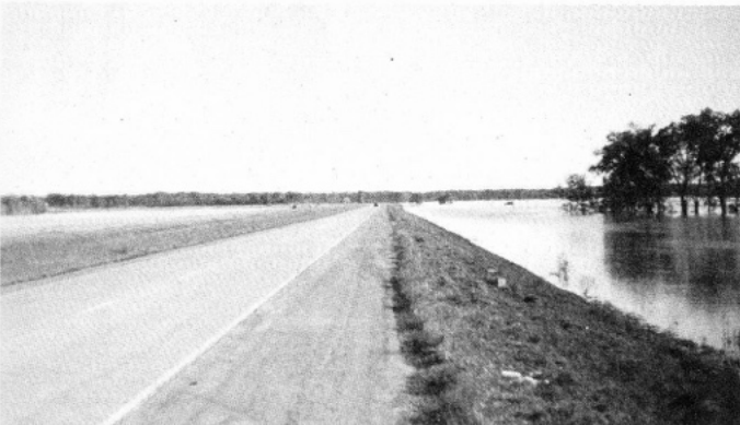
South bound on 71 Highway. Finally letting traffic through.
