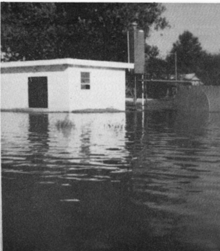
Sand bags kept rising water out of the water plant.
