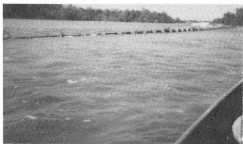
Approach to new bridge on north AA over Osage River.
