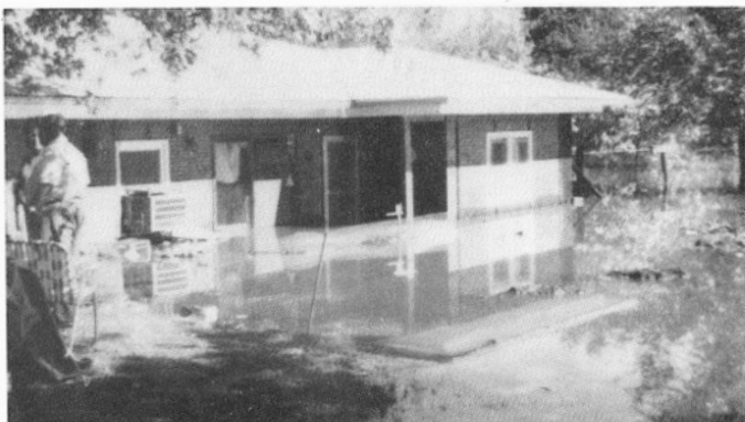
Bob and Ruth Gresham's place. Water was in the house for 3 1/2 days.
