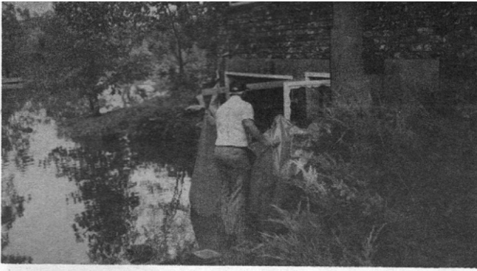
Attempts to use plastic and rows of sandbags failed. M & H Barrow 25-15 Charley Pursley, neighbor, asks if he can help. Later pumped out. Oct. 5, 1986.
