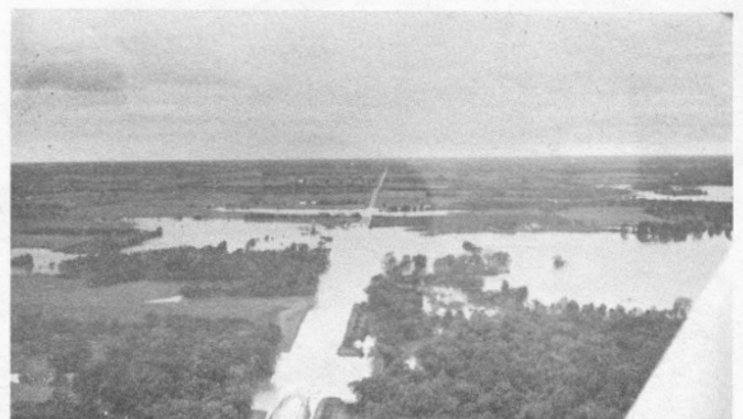
Highway 54 at Deerfield, Mo.
