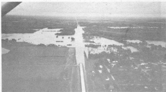
Looking east to west on 54 Highway, Deerfield, Missouri.
