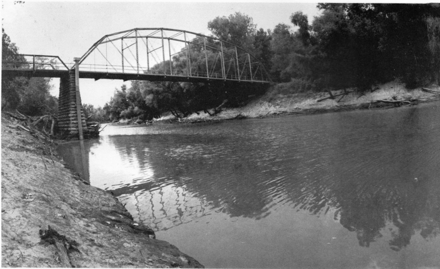
Old bridge north of Schell City.
