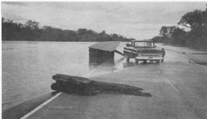
New Highway 54 bridge under water, saving the hog shed.
