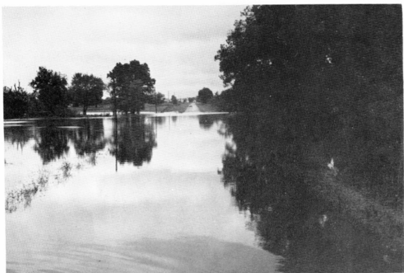
Highway M , north of Compton Junction at Mosley Low Water Branch.
