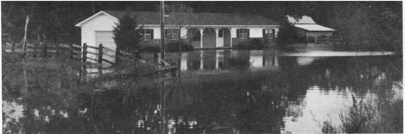
Doug Pettibon's place taken from the Florence Fritz driveway looking down the road towards the pump house bridge over the Marmaton River.
