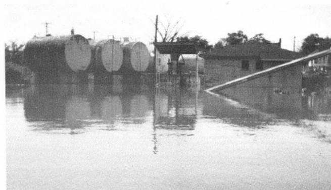
Standard Oil storage tanks on east side of Schell City.
