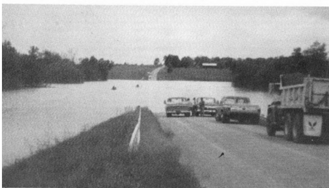
Looking west at Lady Creek crossing M Highway. The bridge was completely under water.
