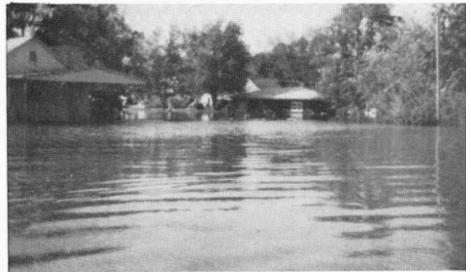
Bob Gresham's earth house in town. Piling up a dike couldn't save it.
