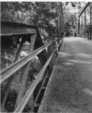
Two historic flood water marks, 1986 is 13' higher than the 1951 mark. This bridge will be torn down and replaced with a larger one.
