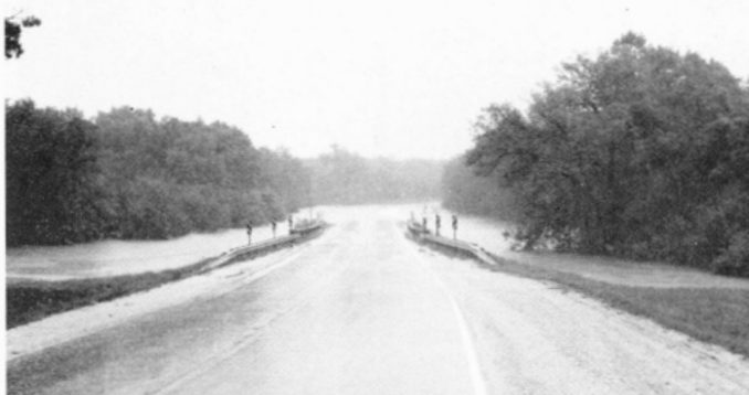
Robinson Branch at 54 Highway east before Clear Creek. Twenty inches of rain. Ja
