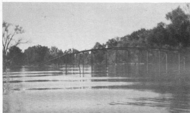
Boater's view of old river bridge. Section 28, Bacon Township.
