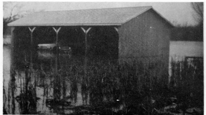
Feb. 27, 1985. This was the highest flood waters had ever come.
